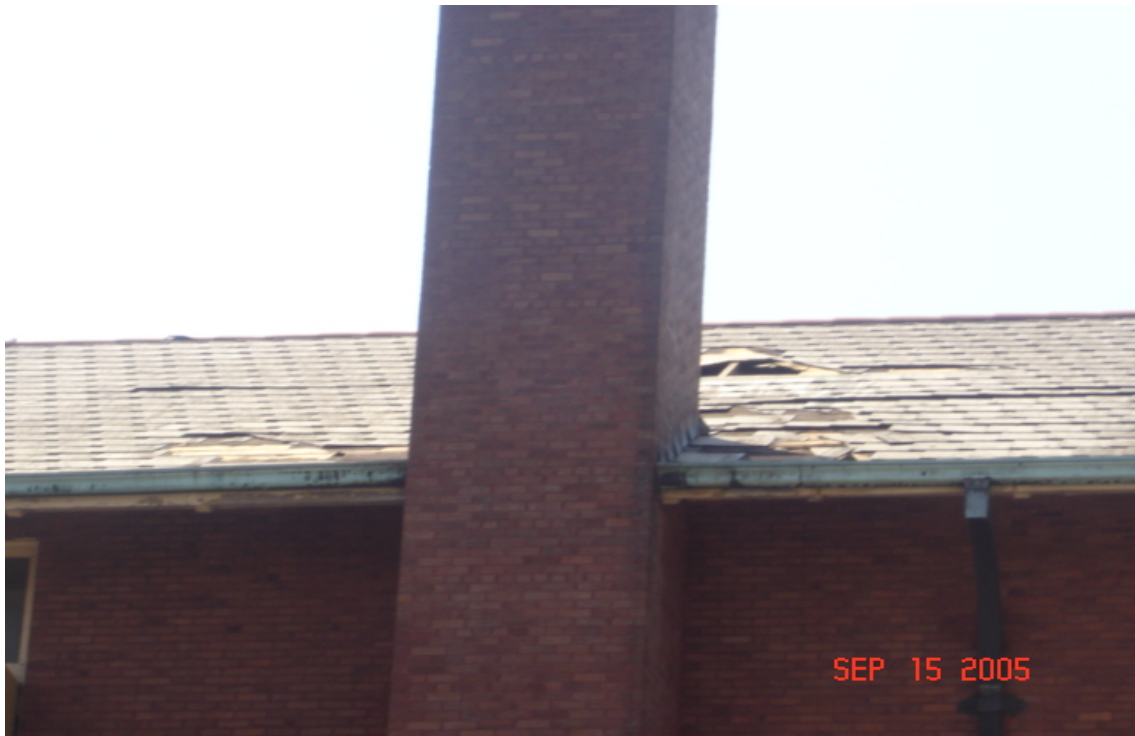
Roof damage
